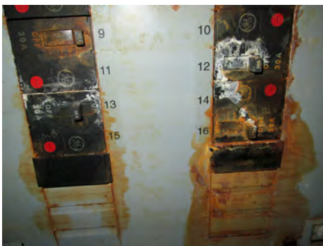
Fig. 1 — Circuit breakers corrode after salt water submersion.
