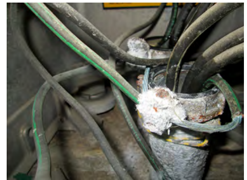
Fig. 6 — Salt residue engulfs a conduit bonding clamp. Corrosion will continue until the salt or clamp is consumed.
