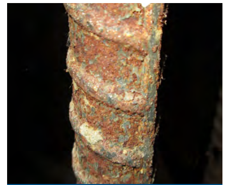
Fig. 9 — Corrosion-induced scaling of this rebar may prevent proper concrete adhesion unless properly cleaned.
