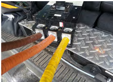
Fig. 5 — The terminals of a newly installed breaker corrode due to saltwater wicking from the existing conductors. The salt water wicked up from the wires terminated at the bottom of the breaker.
