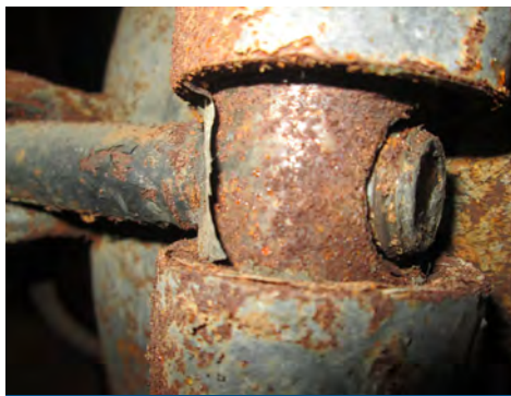
Fig. 8 — Corrosion on the fasteners of this heat exchanger head may make removal difficult.
