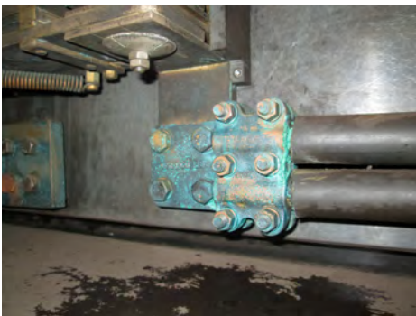
Fig. 4 — This termination point, cleaned twice, continues to corrode due to salt water wicking from the associated conductor.
