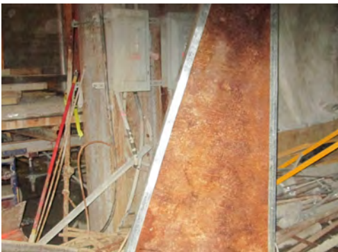
Fig. 7 — Section of ductwork that had been submerged in sea water during Hurricane Sandy. If the surface is not improved, additional drag from the roughened surface will affect system energy consumption.
