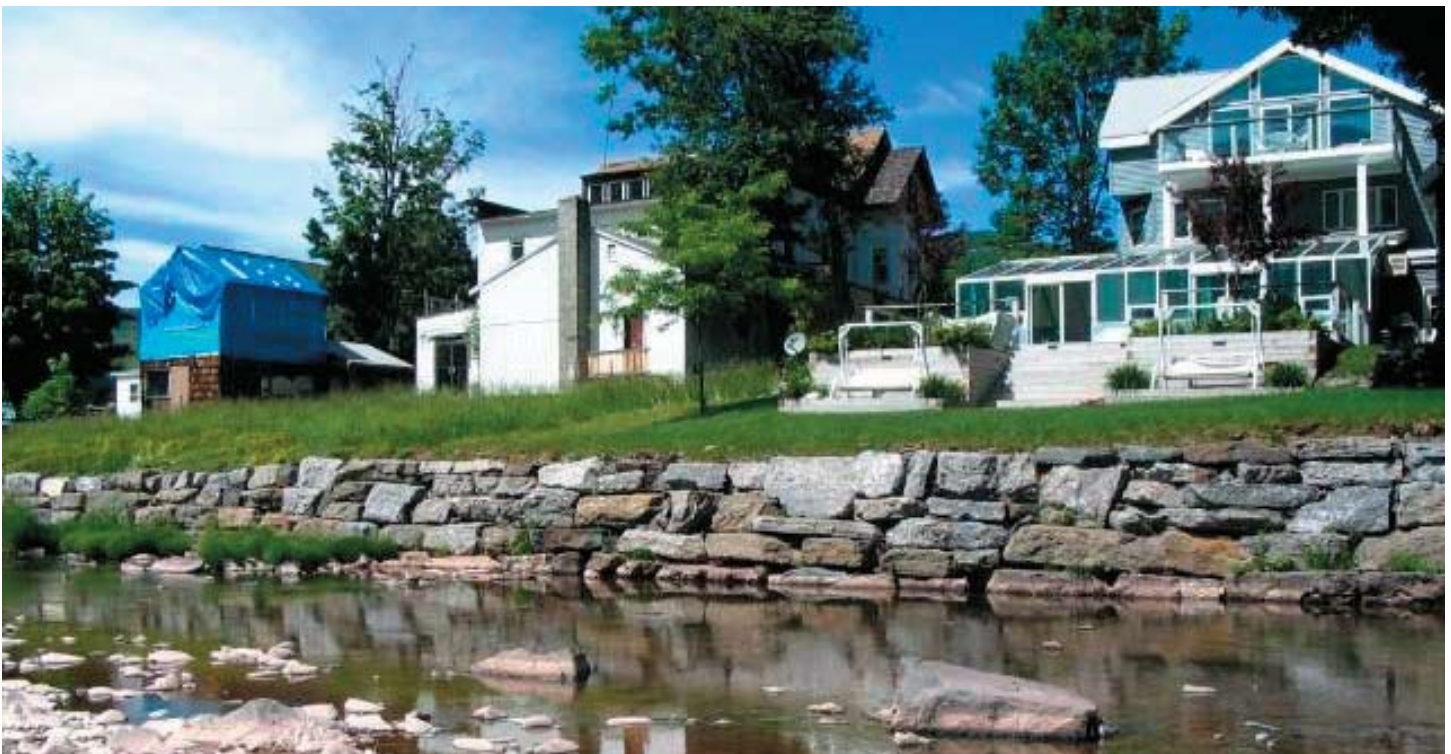
Flood wall protecting homes.
