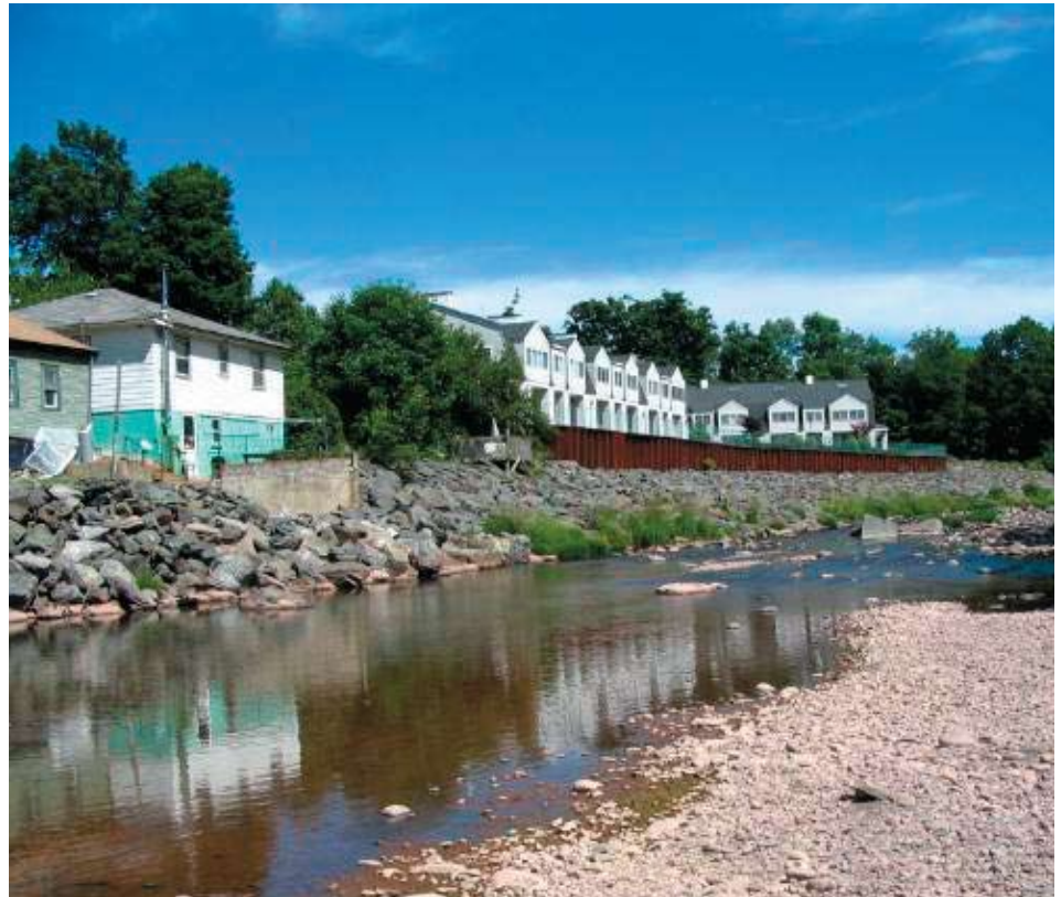
Sheet piling and riprap protecting improved property.
