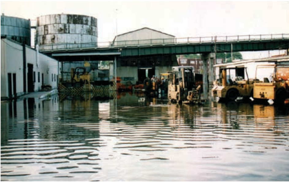
If a declaration is made by a floodplain administrator that a facility is substantially damaged, a determination must be made quickly regarding actions that will need to be taken to make repairs, or whether the facility must be replaced.
